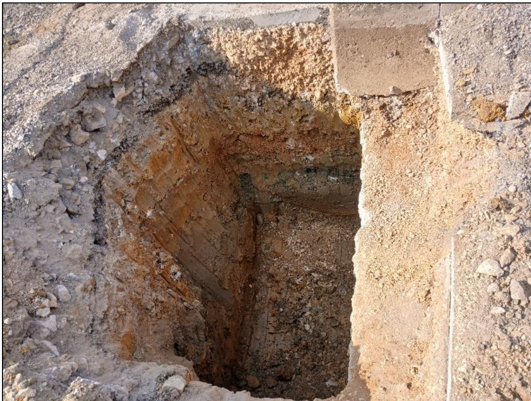
Photo 2: Sinkhole excavated to depth. Stable sidewalls and bottom.
