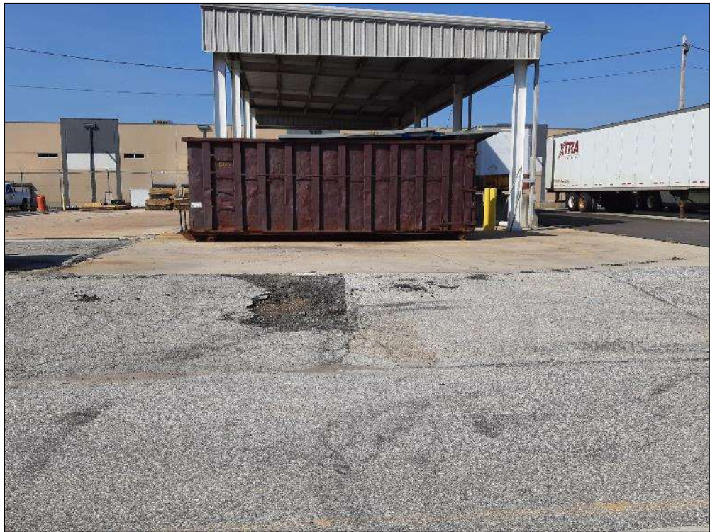
Photo 2: Photo looking west at distressed asphalt located east of the roll box lean to structure. Photo taken March 2024.
