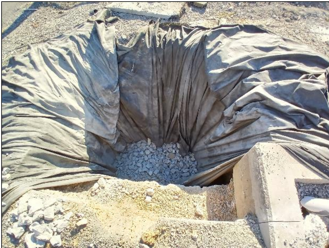
Photo 4: Begin backfill with R4 stone.
