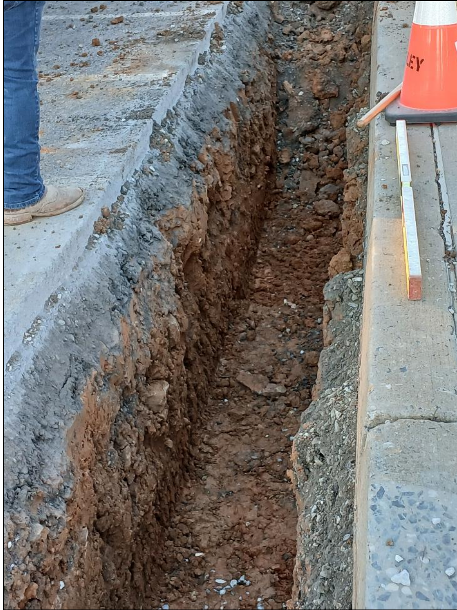
Photo 4: Photo looking west as stormwater utility excavation trench.
