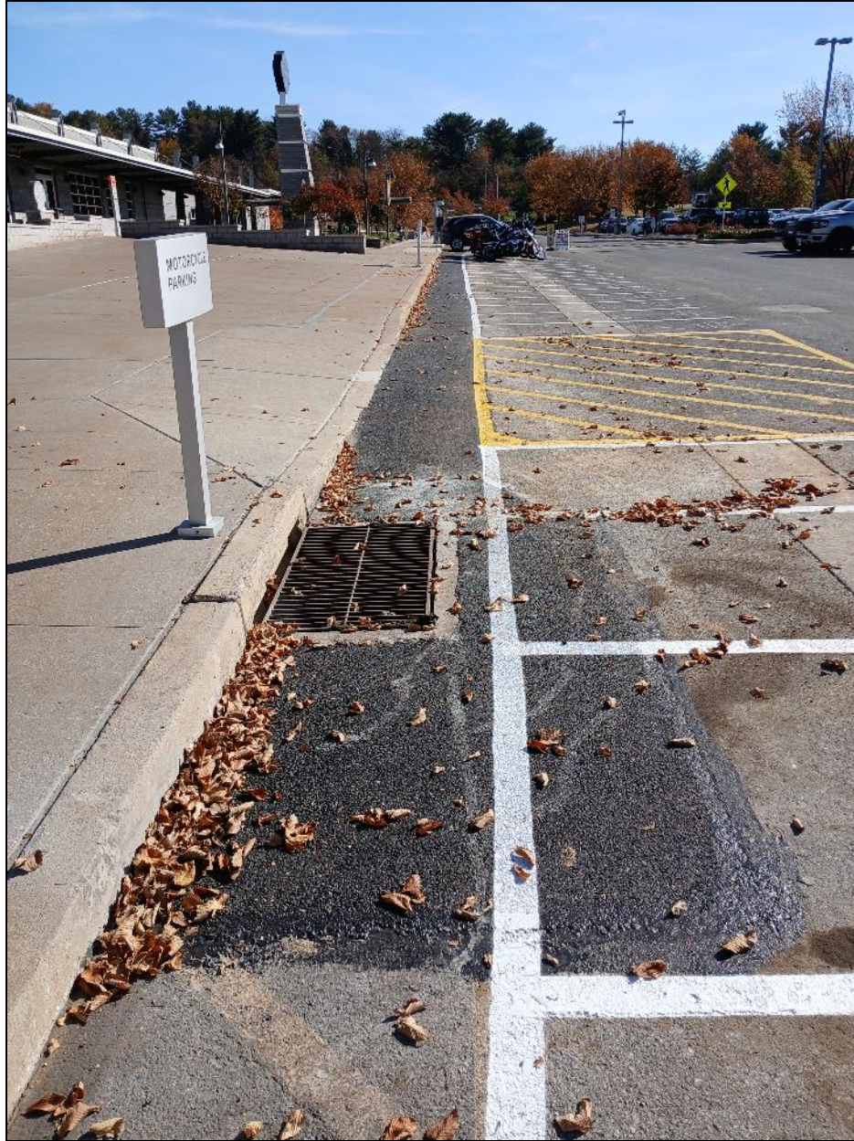
Photo 8: Photo looking east at existing stormwater inlet and piping trench that connect the new inlet. Asphalt is installed and the seams are sealed.
