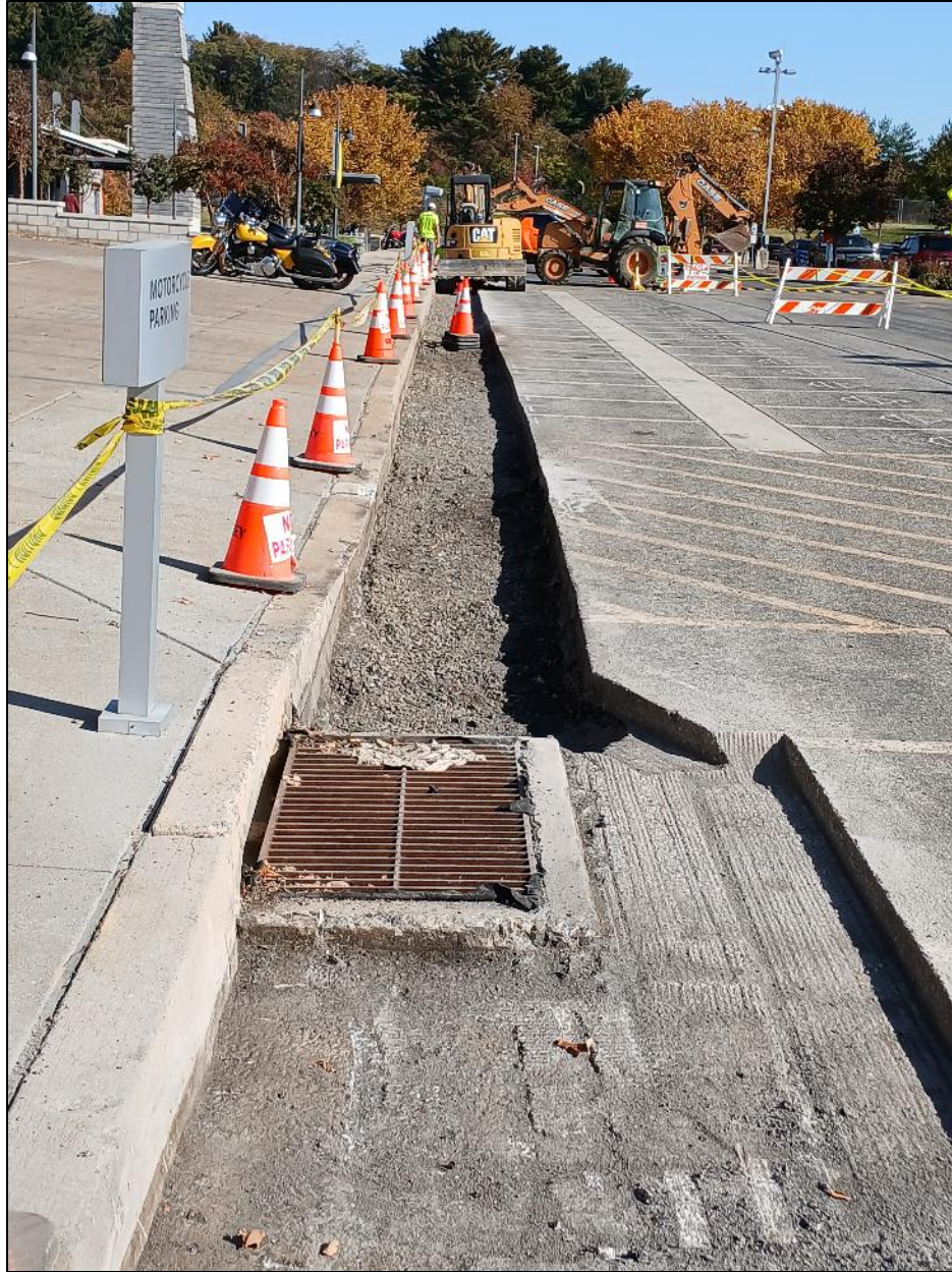
Photo 1: Photo looking east at existing stormwater inlet. Asphalt in utility installation area was milled.
