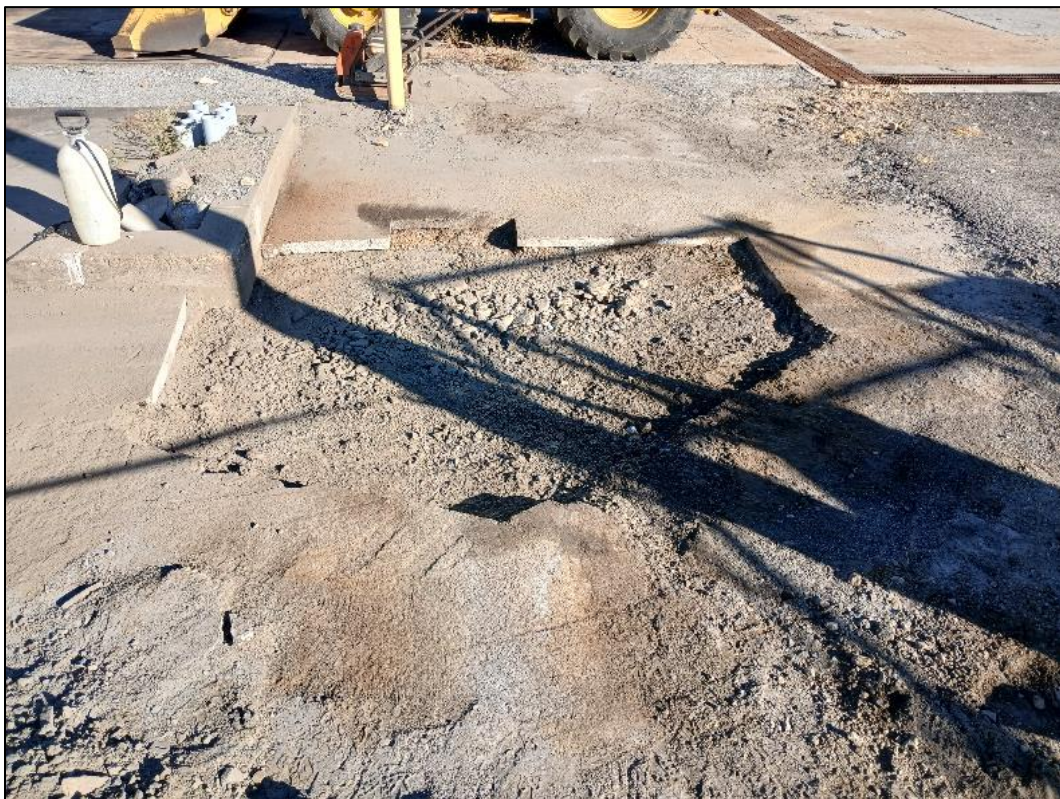
Photo 6: Photo prior installation of asphalt to replace cap.
