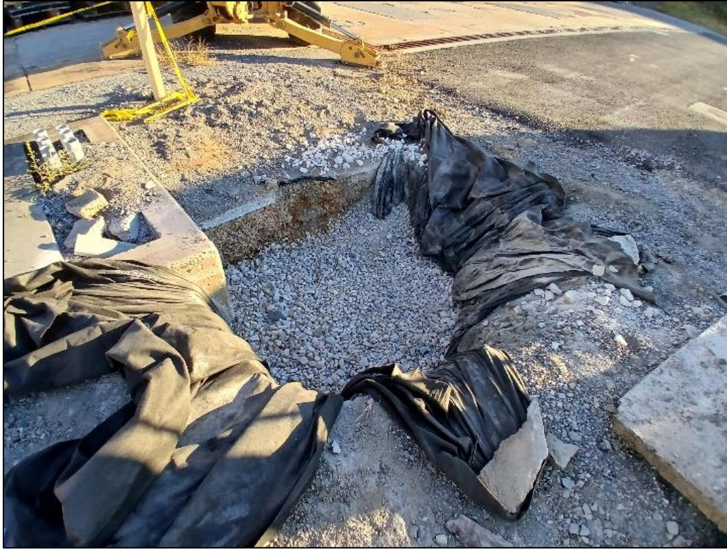
Photo 5: Gravel installed above the R2 stone. Geotextile fabric was folded on top of gravel.
