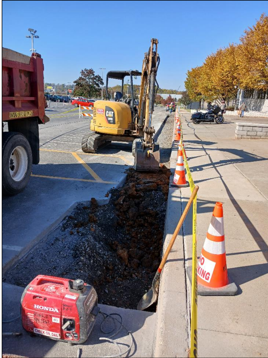
Photo 2: Excavation area where new stormwater inlet will be installed.
