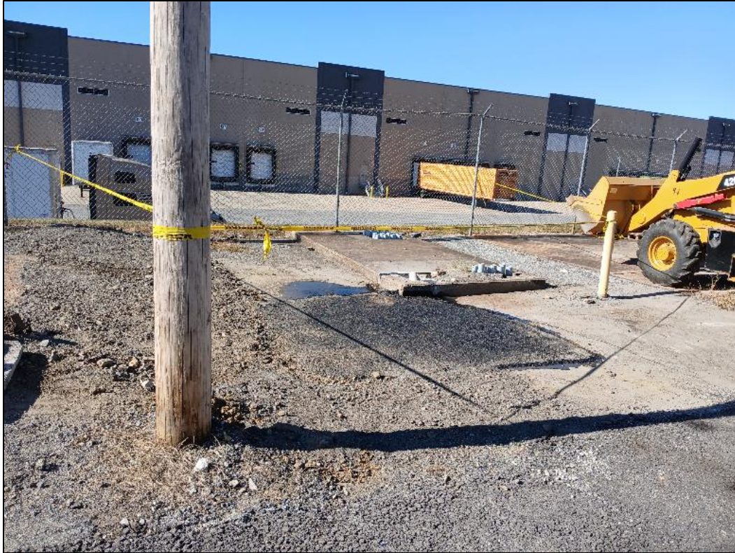
Photo 7: Asphalt cap installed over sinkhole repair area.
