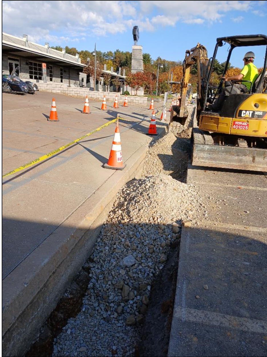
Photo 6: Stone backfill over stormwater installed stormwater pipe.
