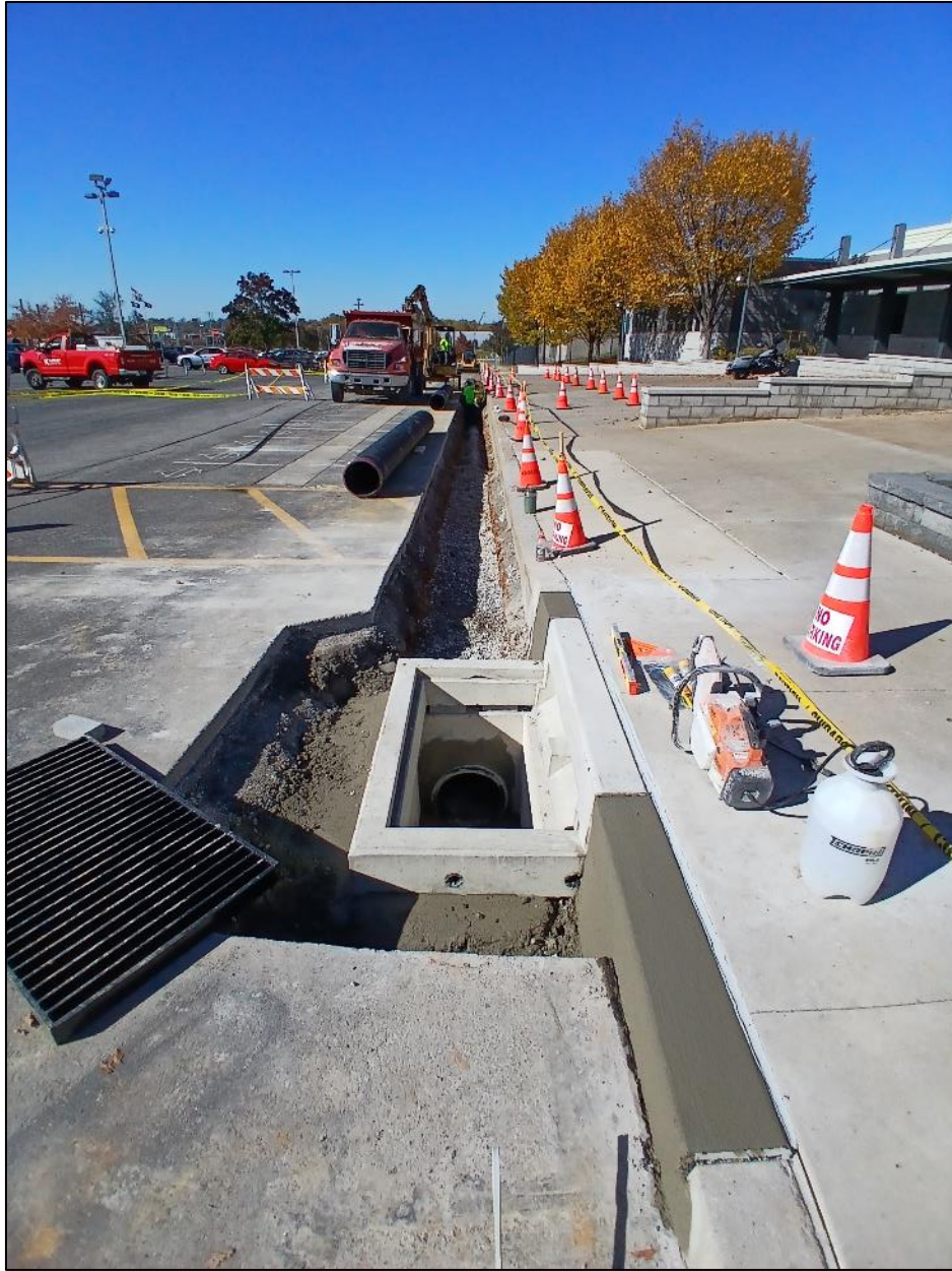
Photo 5: Photo looking west at new stormwater inlet, concrete repairs to sidewalk curb, and stormwater pipe trench.
